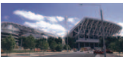
Olympic Stadium, Sydney, Australia
